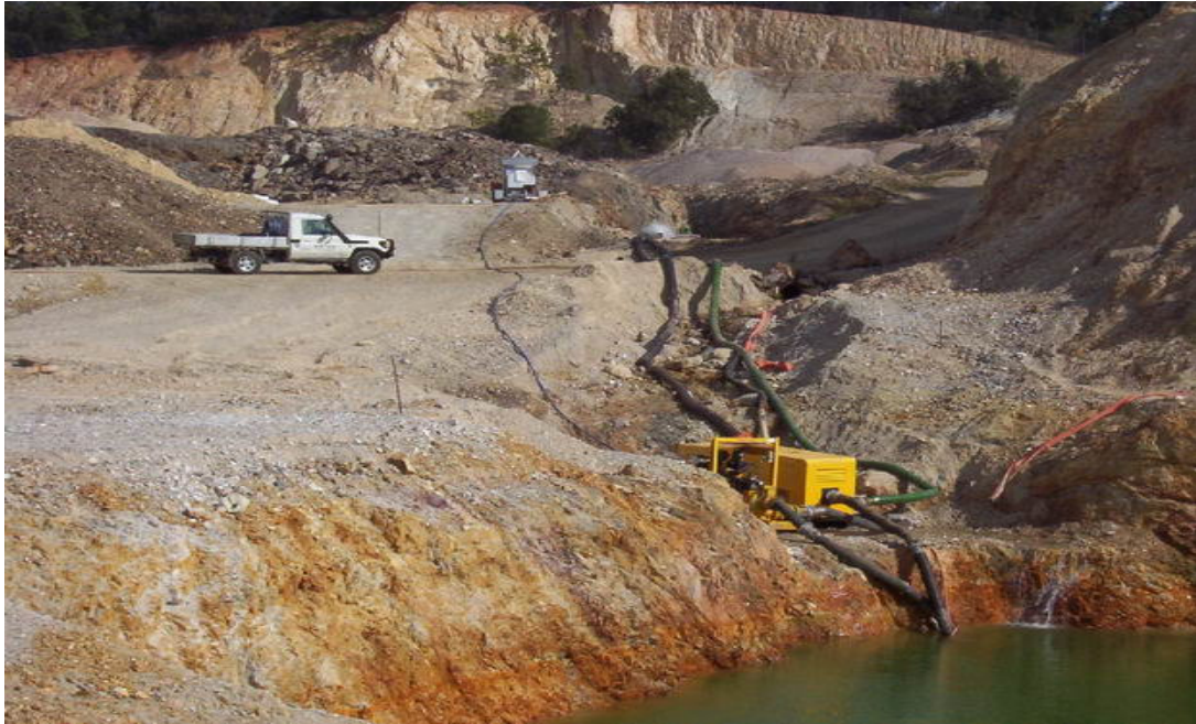
Two 8 inch pumps and CRAB treating fluctuating acidity of pit water.
